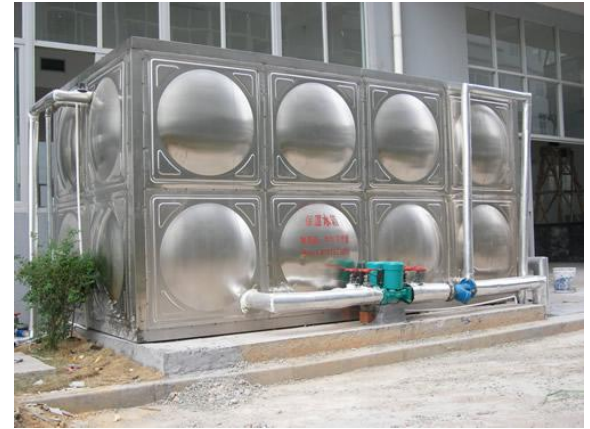
Outside water storage
