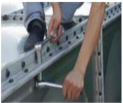
Panels bolt together
