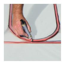
2 Place the cut sheets over the Warmboard panel and tape down the corners. With a permanent marker, trace the tubing pattern, and clearly mark the top and bottom on the stencil. Remove plastic and lay flat next to work area.
