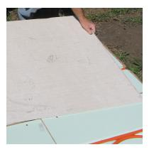
3 Trowel a coat of Thin-Set over the Warmboard panel and place the Backer board over to the appropriate location.
