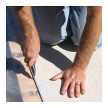
1 Cut the polyethylene to the size of Backer board.
