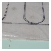
4 Align and tape the stencil down over the Backer board. Pre-drill all safe fastening locations, then remove stencil and fasten as normal.
