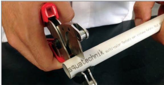
1 – Cut the pipe square using the Safety® system pipe cutter or other suitable tool.
