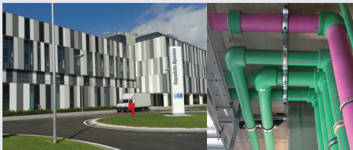
New Hospital Apuano, Massa Carrara, Italy
